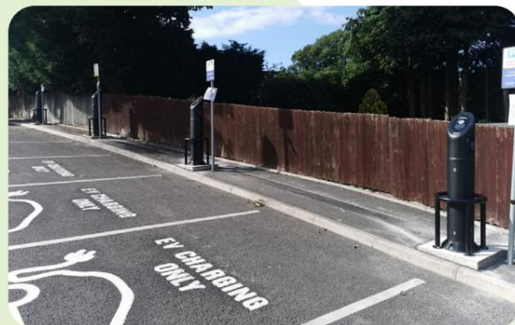
The aim for these car park sites is to install 4 dual socket charge points at each, providing the ability to charge 8 vehicles.
